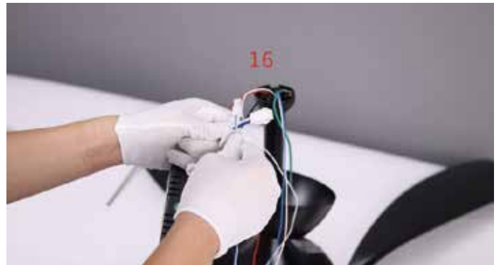
26. Connect the wire from the ceiling fan to the receiver (Blue and White wires)
