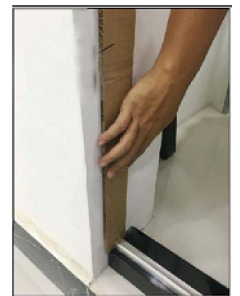
Insert template to bottom door guide.
