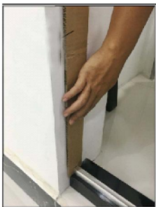
Insert template to bottom door guide.
