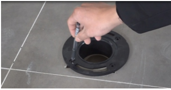
2. Put the flange ring into the drain outlet and mark the screws positions
