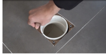
4. Put the screws into the holes
