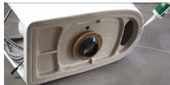
10. Apply some glass glue on the bottom of the toilet (The glass adhesive in the picture needs to be purchased by oneself.)
