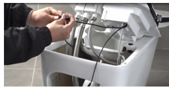
13. Put the toilet seat in the toilet and reconnecting the flexible tube and black wire
