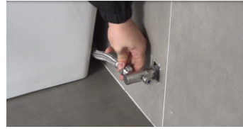
16. Finally connecting the flexible tube to the inlet angle valve
