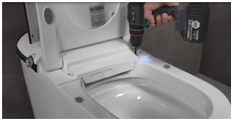
14. Install the screws on the toilet seat and put on the fixing
