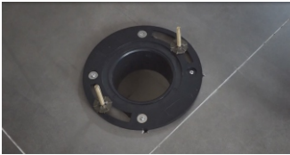
6. Install two long screws as below picture
